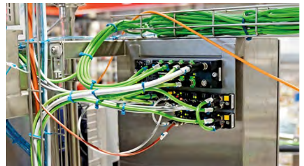
Turck's TBEN-LL-SE-M2 Ethernet switch (above) with eight 100 Mbit and two Gbit ports for fast and secure data transmission in the machine
