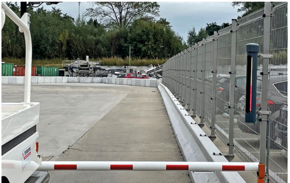
The light points on the WLS27 LED strip visualize a timer that counts down the driver's waiting time
