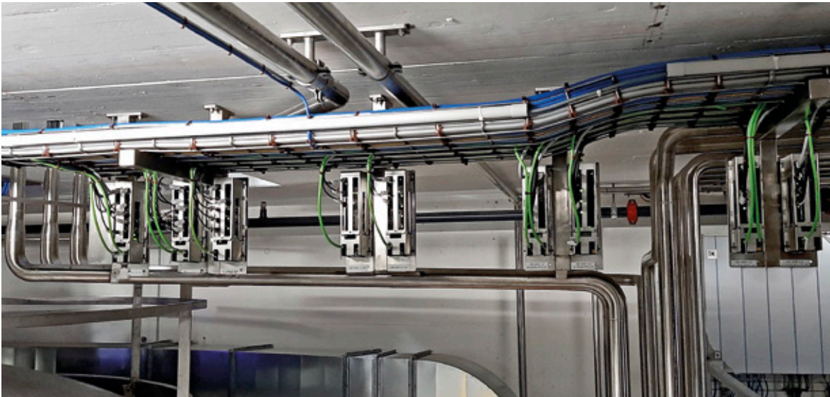
The TBEN I/O block modules are installed under the cable trays in ATEX protective housings to save space
