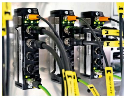
Turck's TBEN RFID interfaces with IP67 protection are screwed onto a metal panel in a cabinet-free installation in the warehouse
