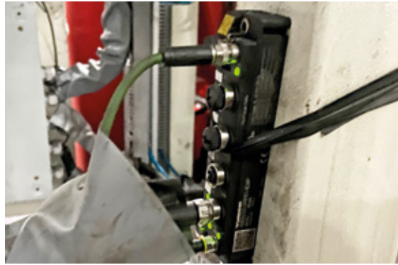
With its 16 kilobyte data buffer, Turck's TBEN S RFID module offers impressive performance
