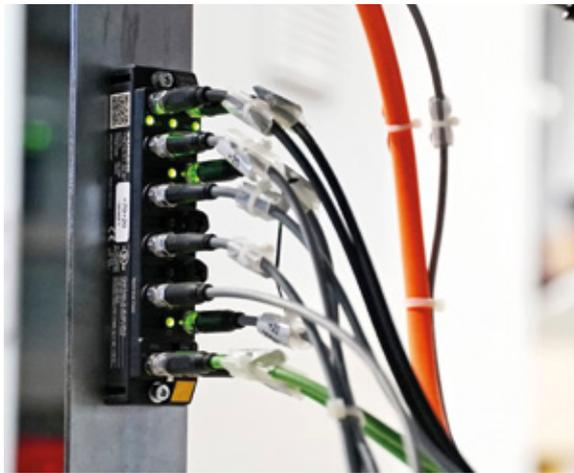
Turck's I/O components with decentralized control logic move the required intelligence to the direct environment of the conveying line
