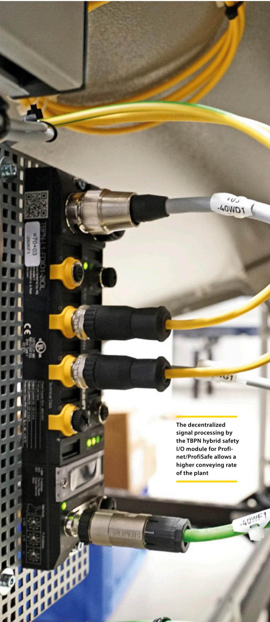
The decentralized signal processing by the TBPEN hybrid safety I/O module for Profinet/ProfiSafe allows a higher conveying rate of the plant
