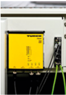
Fast cabling, easy installation: The robust PSU67 power supply provides all required voltages directly on site
