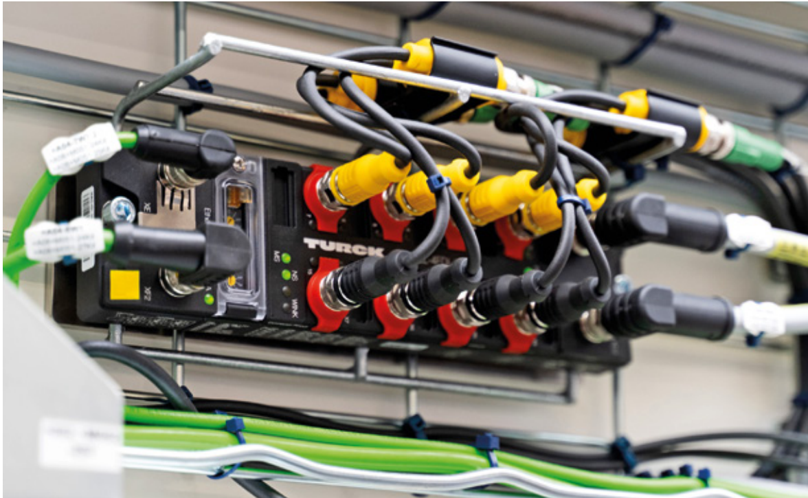
TURCK's consistent multi-protocol strategy also pays off in the field of safety technology, as demonstrated here by the TBIP safety module for EtherNet/IP and CIP Safety
